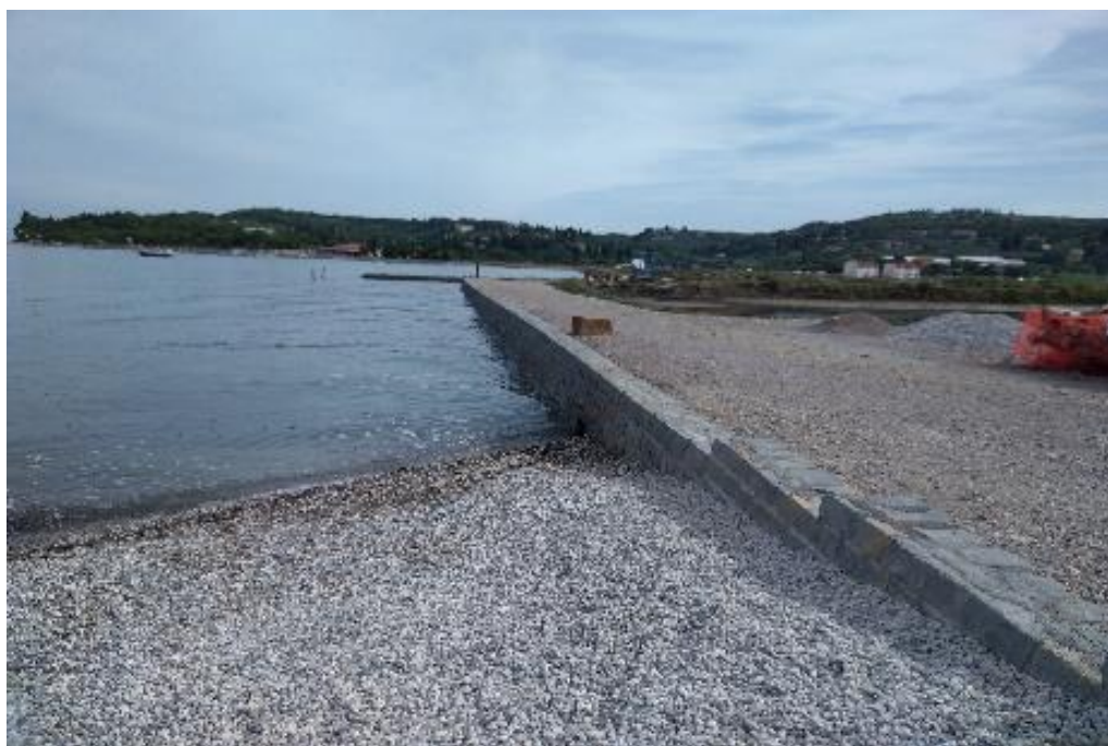
Figure 8: Stjuža Strunjan. Case of artificial coastline that is concrete coated (Coastline section with ASCODE: 2) (Photo: IWRS, 2019).
