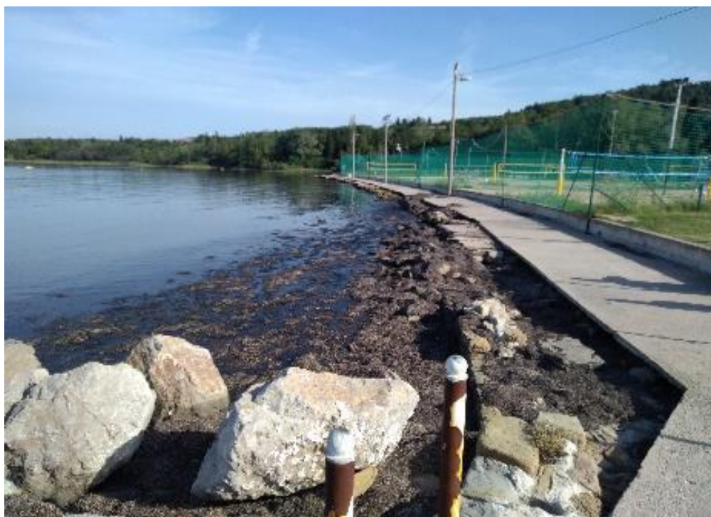
Figure 4: Bay of St. Katarina. Case of artificial coastline that is concrete hardened (Coastline section with ASCODE: 2) (Photo: IWRS, 2019).
