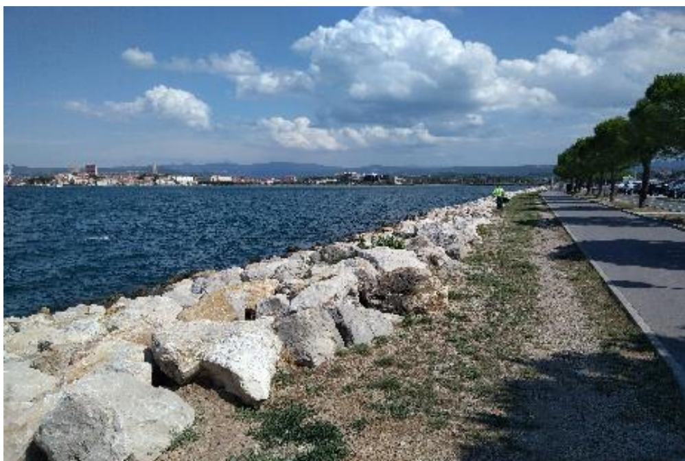
Figure 7: Coastal road from Koper to Izola. Case of artificial coastline with stone blocks (Coastline section with ASCODE: 2) (Photo: IWRS, 2019).
