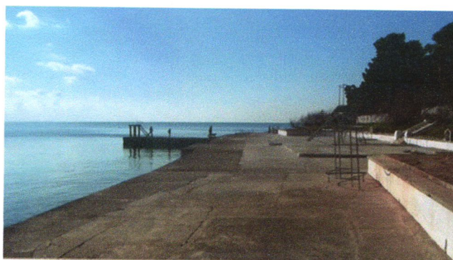
Figure 7: Concrete and leveled the rocky coast – “Valkane” beach, city of Pula (Photo: Latinka Janjanin, 2012.)
