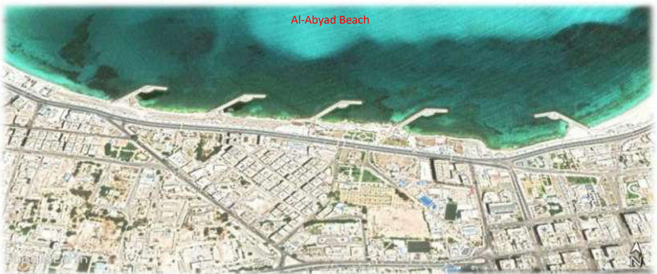
Fig (22): Recent Beach Protection Projects
