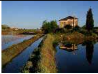
Photo 106: Saltpan house and channel
