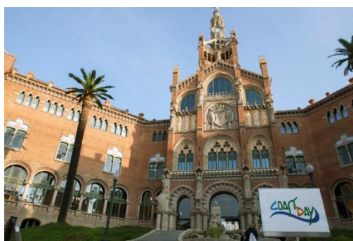
Sant Pau Art Nouveau Site, main entrance
