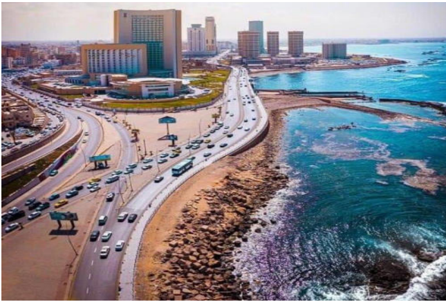
Figure No. (16): Tripoli Sea Road Revetments
