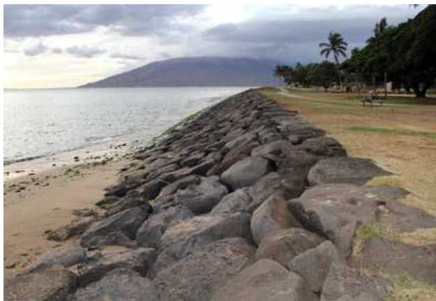
Slika 6.18: Primjeri zaštitnih građevina na obalnoj crti (Izvor: Envirostruct Services, http://estruct.com.au/waterways/revetment-walls/coastal-protection/ )
