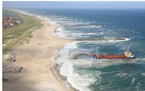
Slika 6.10: Obnavljanje plaže (Izvor: http://eng.kyst.dk/coastal-protection-on-the-west-coast-of-jutland.html )
