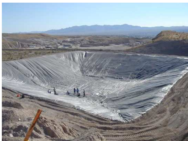
Slika 6.32: Retencija u gradnji. (Izvor: http://www.royalflushservices.com/excavating-contractor-eugene-oregon/ )
