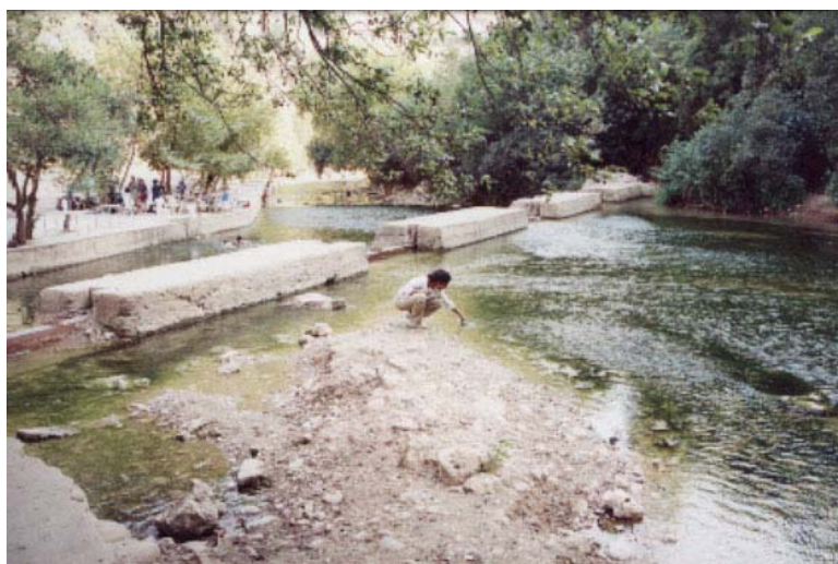
Photograph 6.2. Upper Dam on the Damour River
