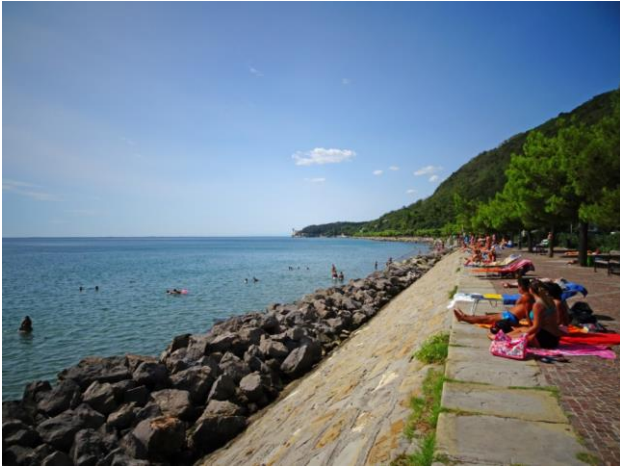
Figure 31. The seawall between Miramare and Trieste (Photo: Enzo Pranzini)
