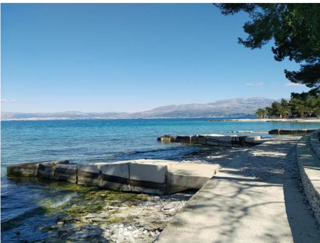
Figure 35. Groynes in Misano, Italy (above) and Supetar, Croatia (below) (Photos: Enzo Pranzini and Ivan Sekovski)
