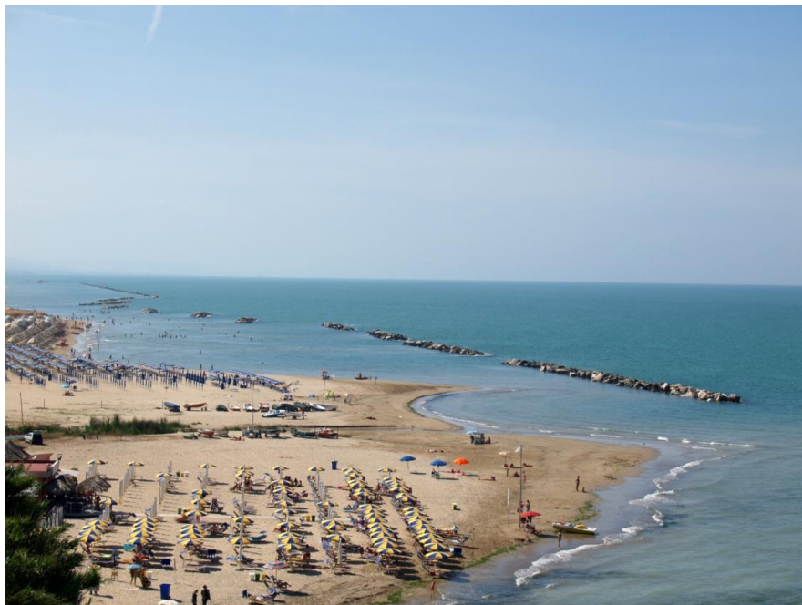
Figure 34. Breakwaters on Torre Mucchia beach, Italy (Photo: Enzo Pranzini)
