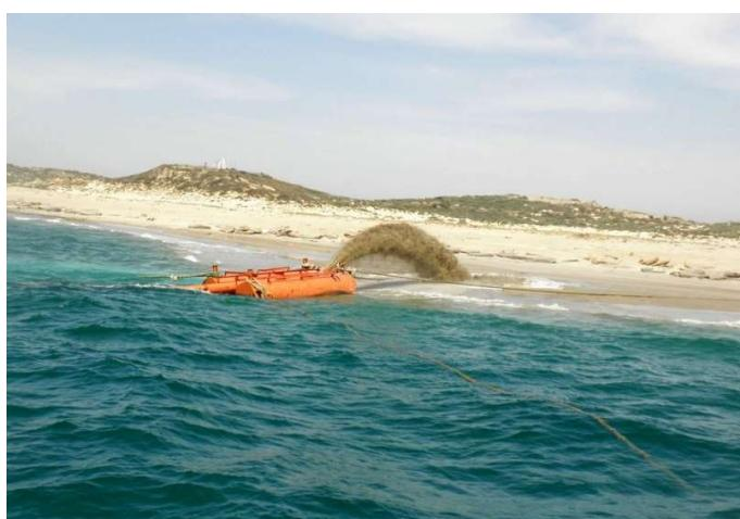
**Figure 36.** Nourishment rainbowing operation via discharge pipe.
