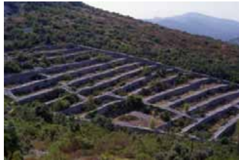
Photo D117: Renewed stone terraces in the island of Korčula
