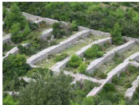
Photos E13 and E14: It took an agricultural labourer a period of fifty years to build drystone walls up to 1 m thickness. Although this example of terraces is exceptionally valuable, they fall into decay due to the absence of heirs.
