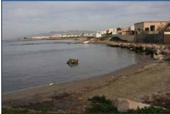
Photo B34: The effect of beach erosion: housing units practically on the water's edge as a result of accelerated erosion.
