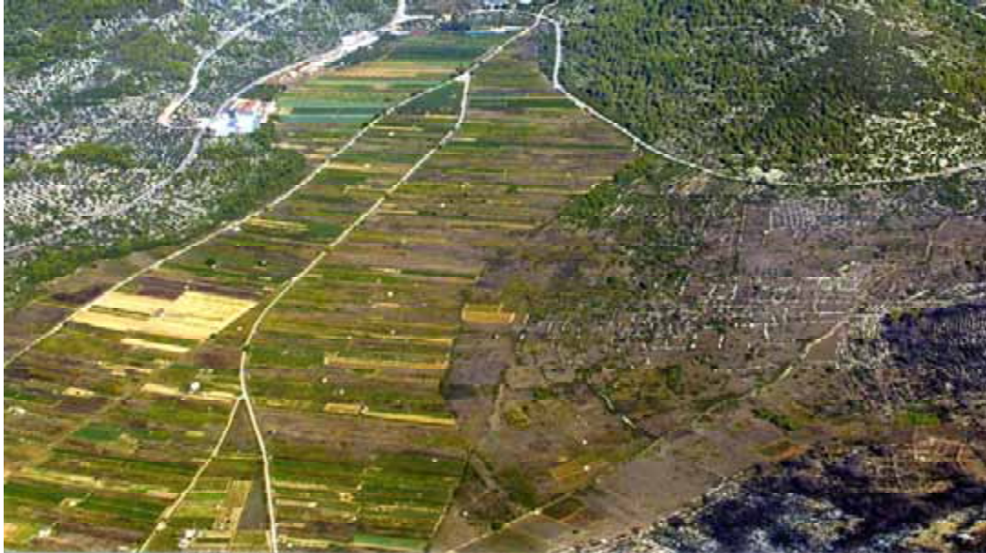
Photo E27: Existing situation in 2005
