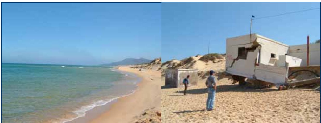
Photo B21: The effects of accelerated beach erosion at Zouaraa, leading to strandline retreat and loss of sand material throughout the system, including beach and dunes.
