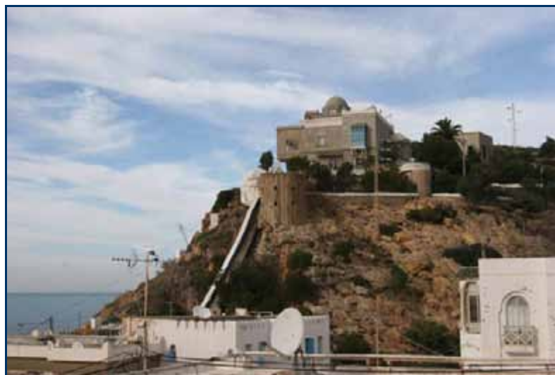
Photo B33: Extensive use of concrete in coastal localities near Korbus.
