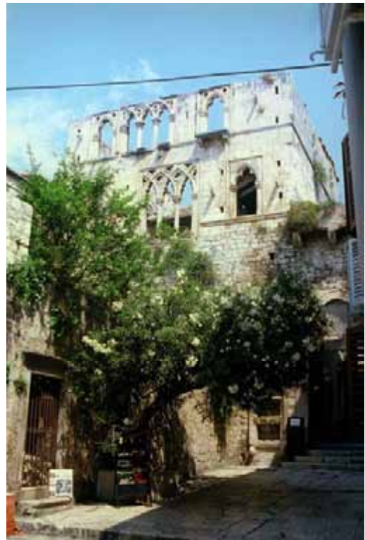
Photo D15: Abandoned villa in Hvar, Croatia
