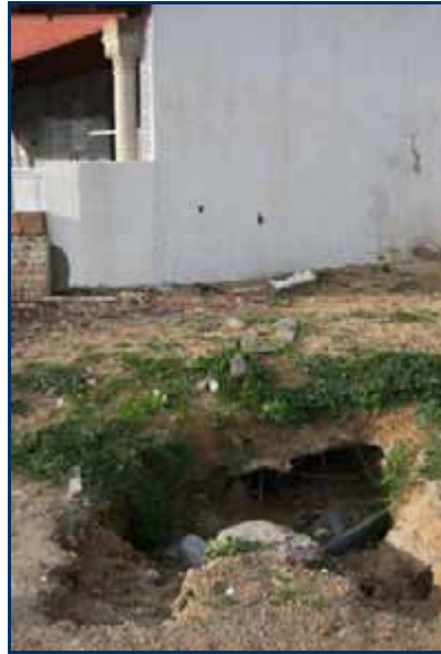
Photo B31: What future? Erosion collapse and instability of sandy substrates, where housing units were constructed on beaches at Soliman.
